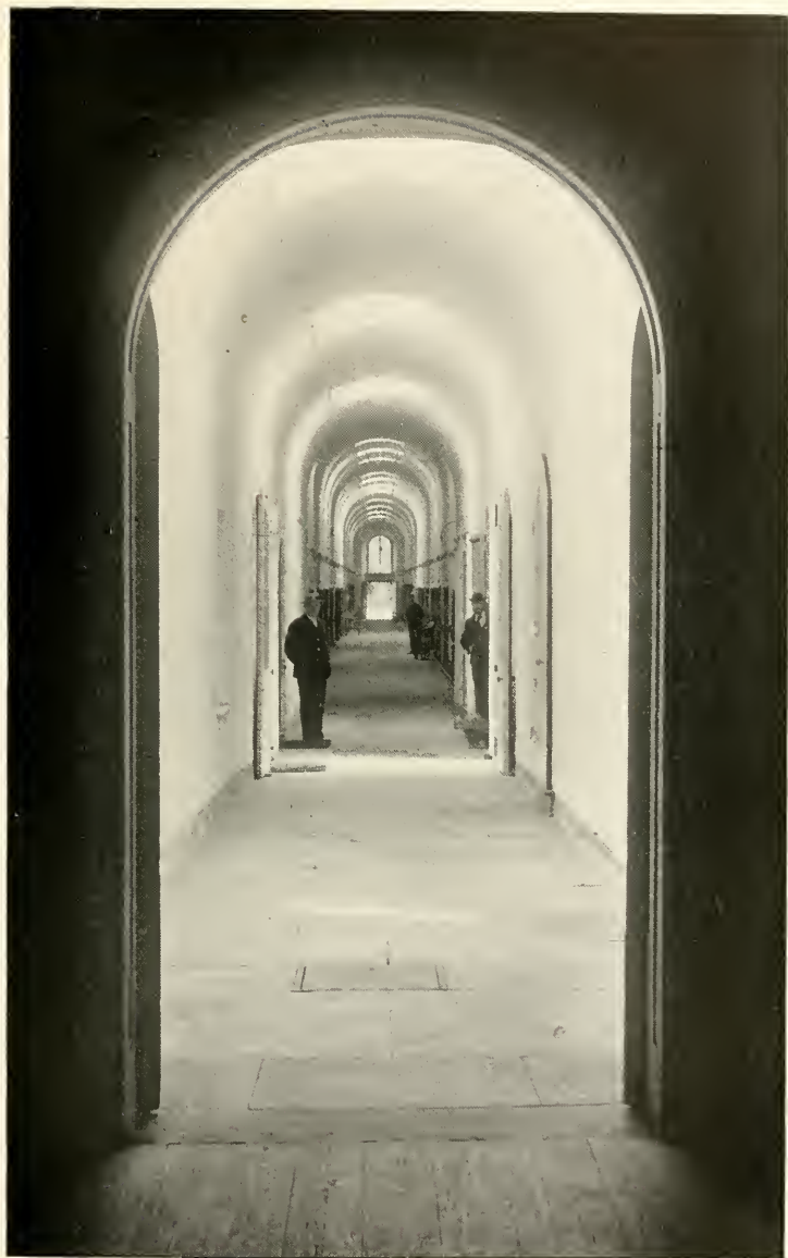
Third Block—368 feet long, 10 ft. wide, 16 ft. high—20 Rooms, 12x7 ft. 6 in., 14 ft. high—12 Rooms, 25x8 ft., 14 ft. high—8 Rooms, 20x17 ft., 14 ft. high—Eastern State Penitentiary.
